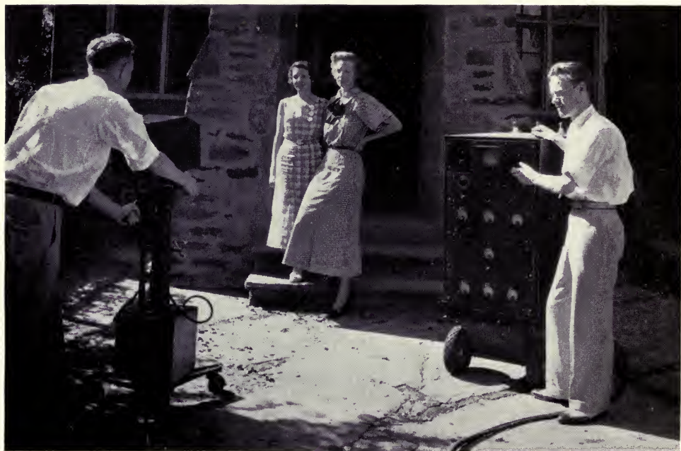
Farnsworth operating his first portable television transmitter unit
